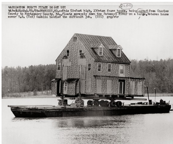
Gordon Matta-Clark, « Untitled / This 50-foot high, 130-ton frame house, being moved from Charles County to Montgomery County, Md., floats serenely down the Patuxent River on a large, Veteran house mover. », 1974.
